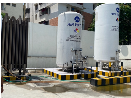
Figure 28: LMO container in a tertiary care center
