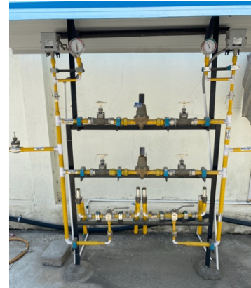
Figure 30: Gas control chain
